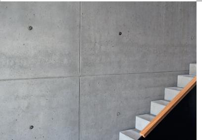
The innovative closure visually enhances every exposed concrete wall. The packers are tensioned in the openings with a hexagon via the pan-head screw - even the overhead insertion in ceilings works uncomplicatedly.
